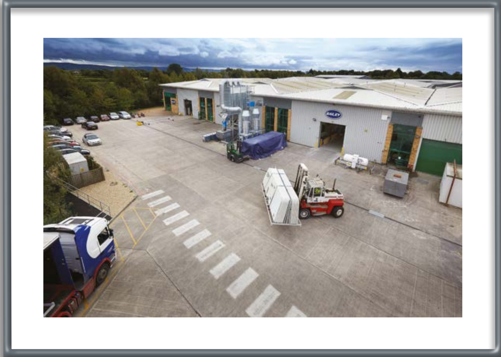
The Large Panel Laminating Plant was the next department to relocate to its own premises in Clevedon, North Somerset. The new site, measuring 3,250+ sq.m. in size, accommodates four state of the art laminating lines, which can produce over 1,500 bodysell panels in just one week.
