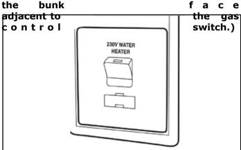
The water temperature cannot be selected; temperature is automatically limited to 70°C. For a faster heating up the appliance can be simultaneously operated with gas and electrical power.
